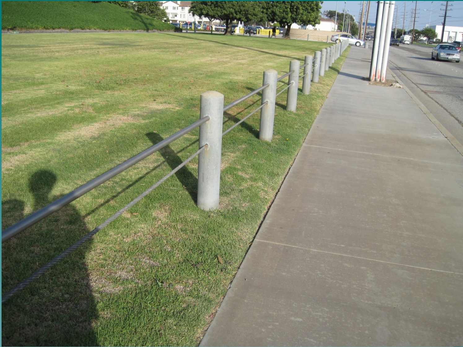
Guard rail and power pole to be relocate at FAA building
