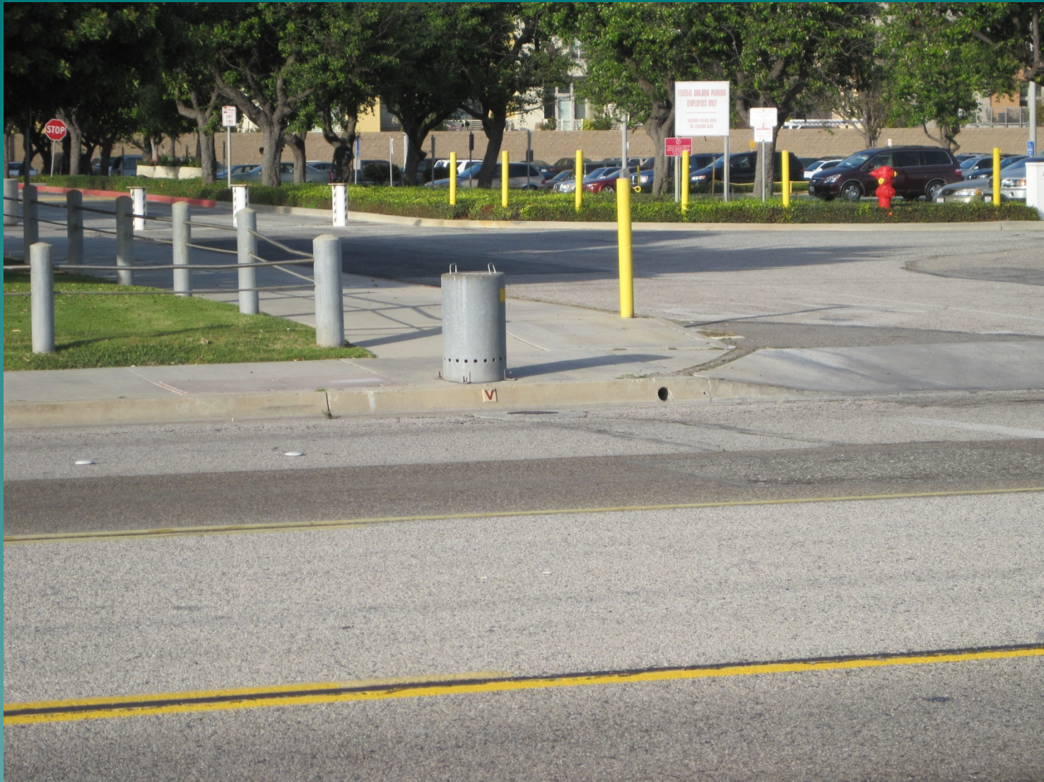
Reclaimed water vault and vent to be relocated at FAA building
