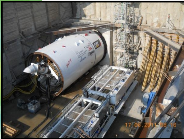
ENTRY SHAFT (JWPCP)
