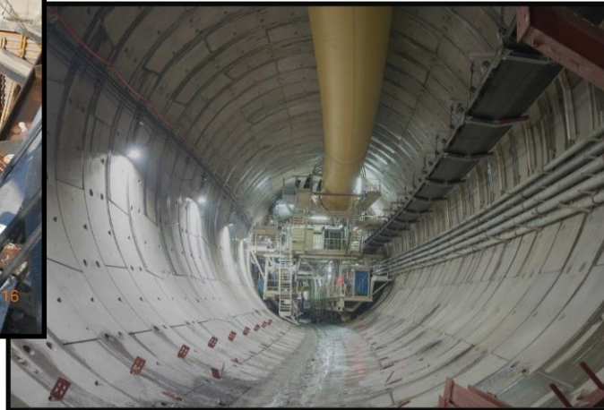
TUNNEL BUILT AS YOU GO (4 years to construct)
