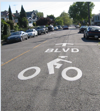
Bicycle Boulevard Marking Berkeley, CA
