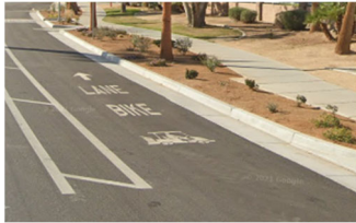
Example of a Class II+ NEV lane from La Quinta, CA with custom NEV marking
