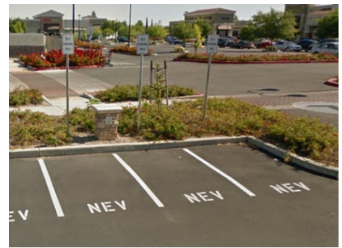
Public NEV parking and charging, Lincoln, CA.
