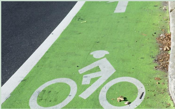
Green Colored Pavement in California had Interim Approval, but is now part of the most recent CA MUTCD
