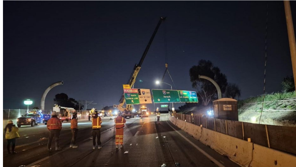
Segment 1: Overhead signage removal on the eastbound I-105 near Vermont Av
