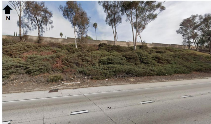
Typical I-105 retaining wall construction area
