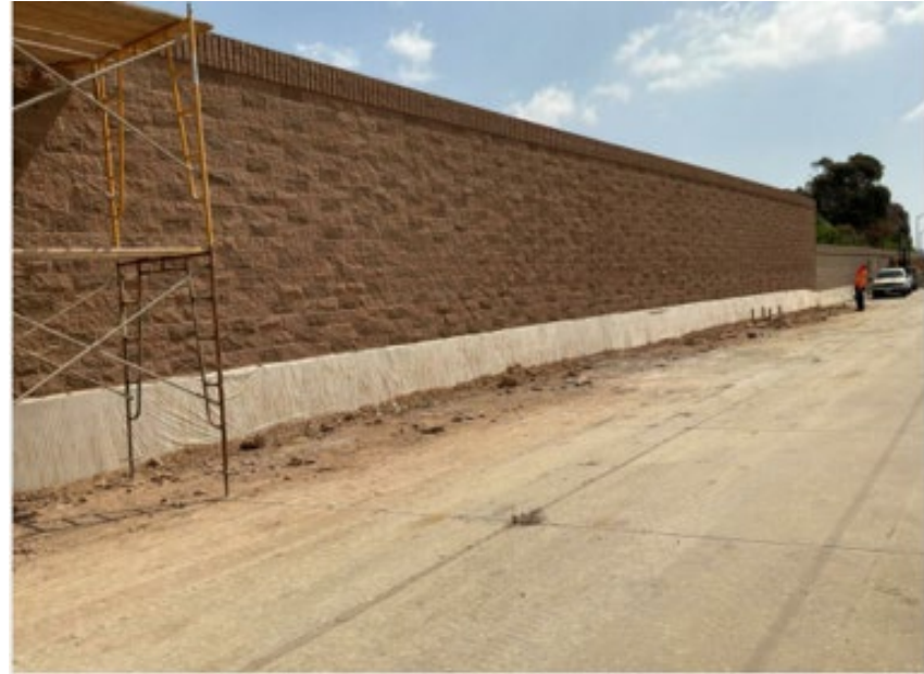
New sound wall: Westbound I-105 in Inglewood
