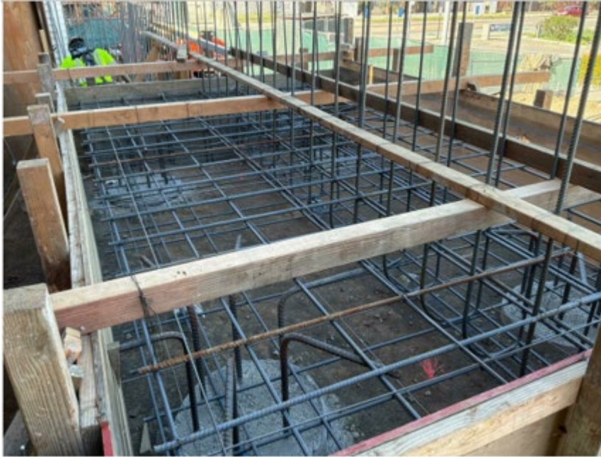
Westbound Avalon BI undercrossing abutment footing
