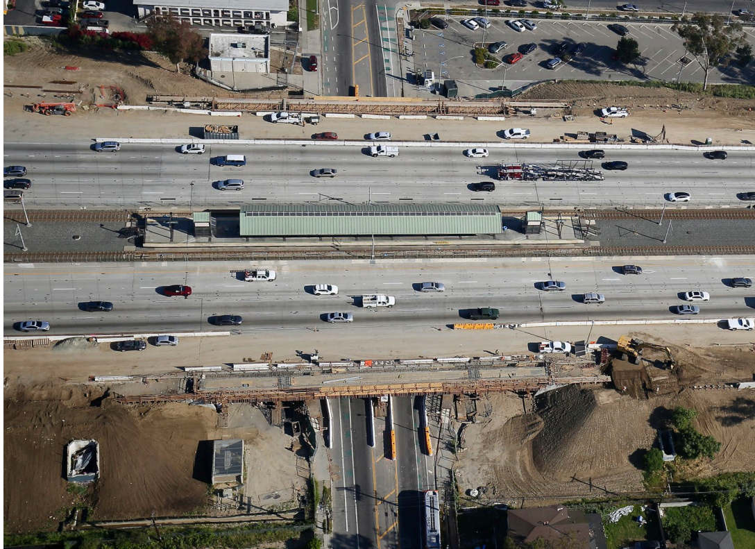
Avalon BI undercrossing construction
