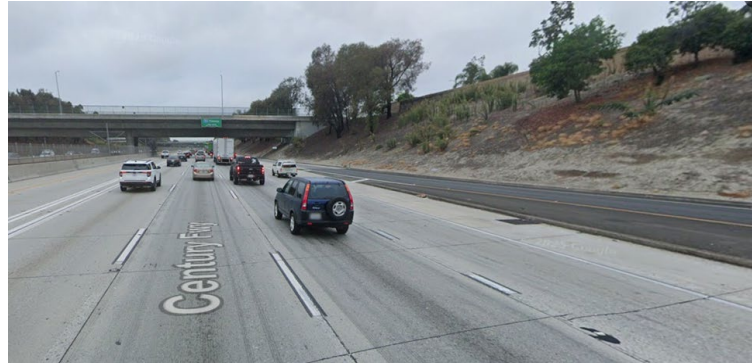
Typical I-105 retaining wall construction area
