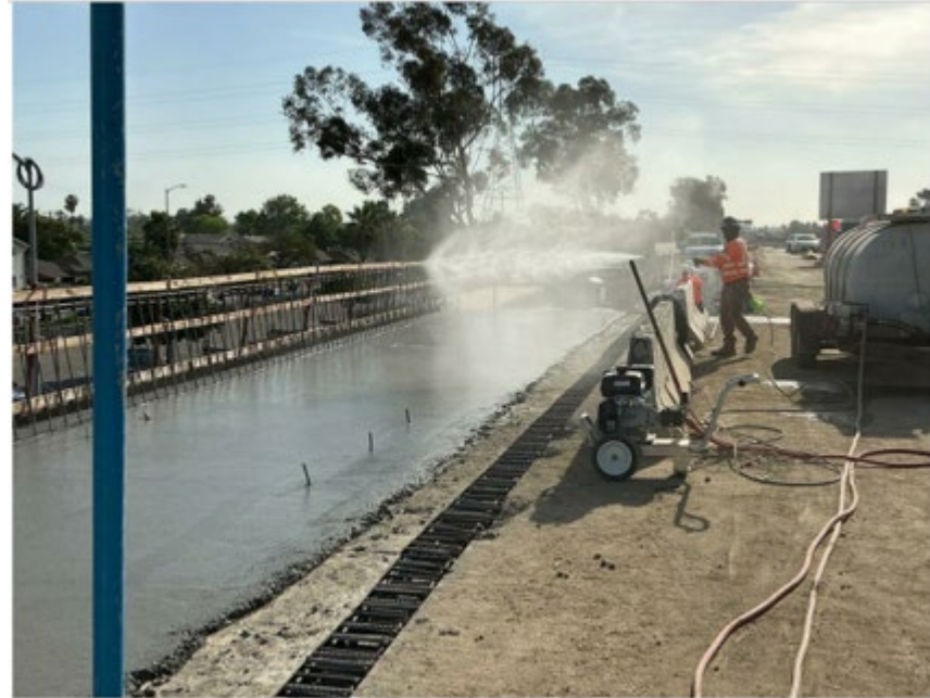
Westbound Avalon BI undercrossing concrete work
