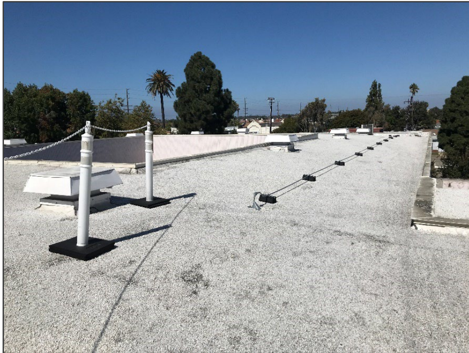
Figure 22 Existing Built-Up Roof with Gravels
