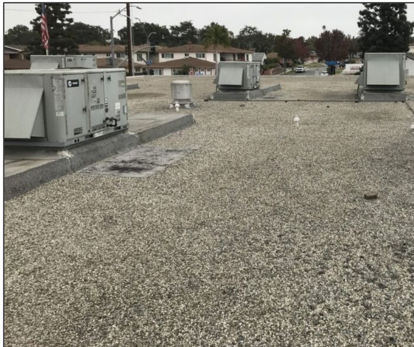
Figure 13 Existing Built up Roof with Gravel Coating on Top
