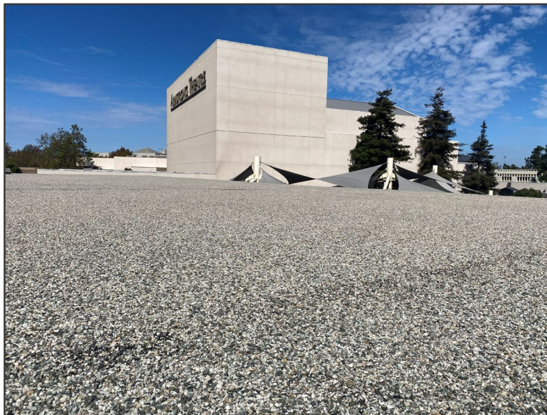
Figure 38 Existing Built up Roof with Gravel Coating on Top
