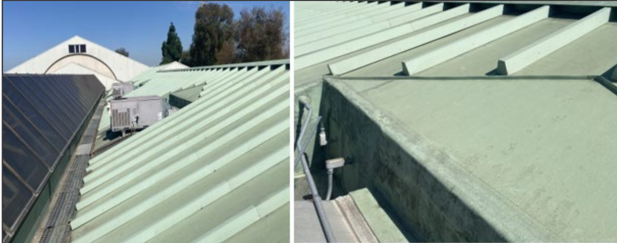
Figure 2 Existing Green Metal Roof
