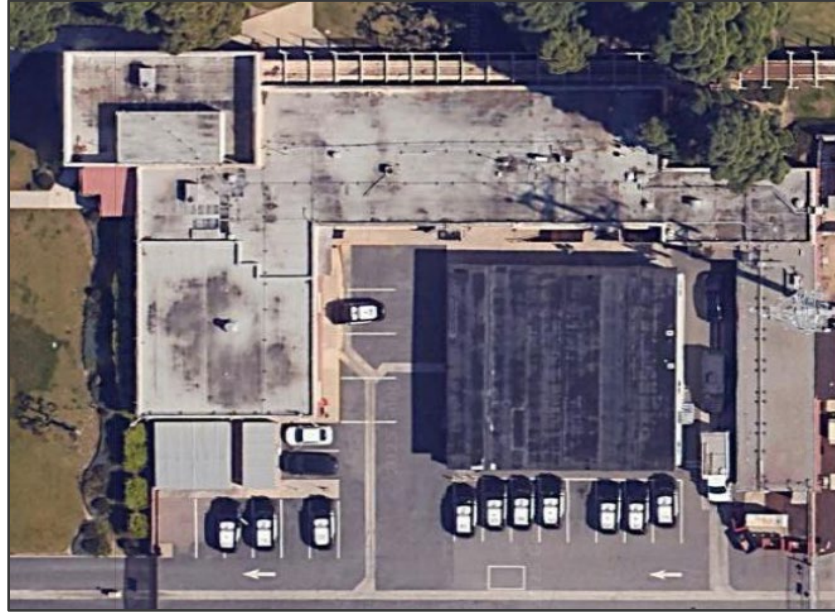
Figure 4 Aerial View of Gardena Police Department
