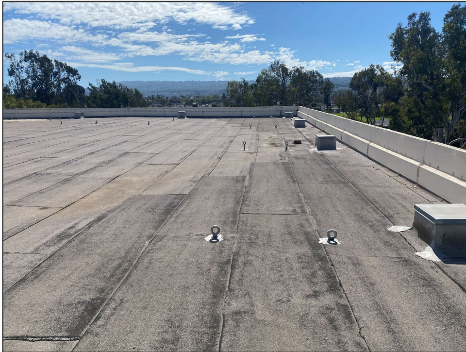
Figure 35 Existing Asphalt Membrane Roof
