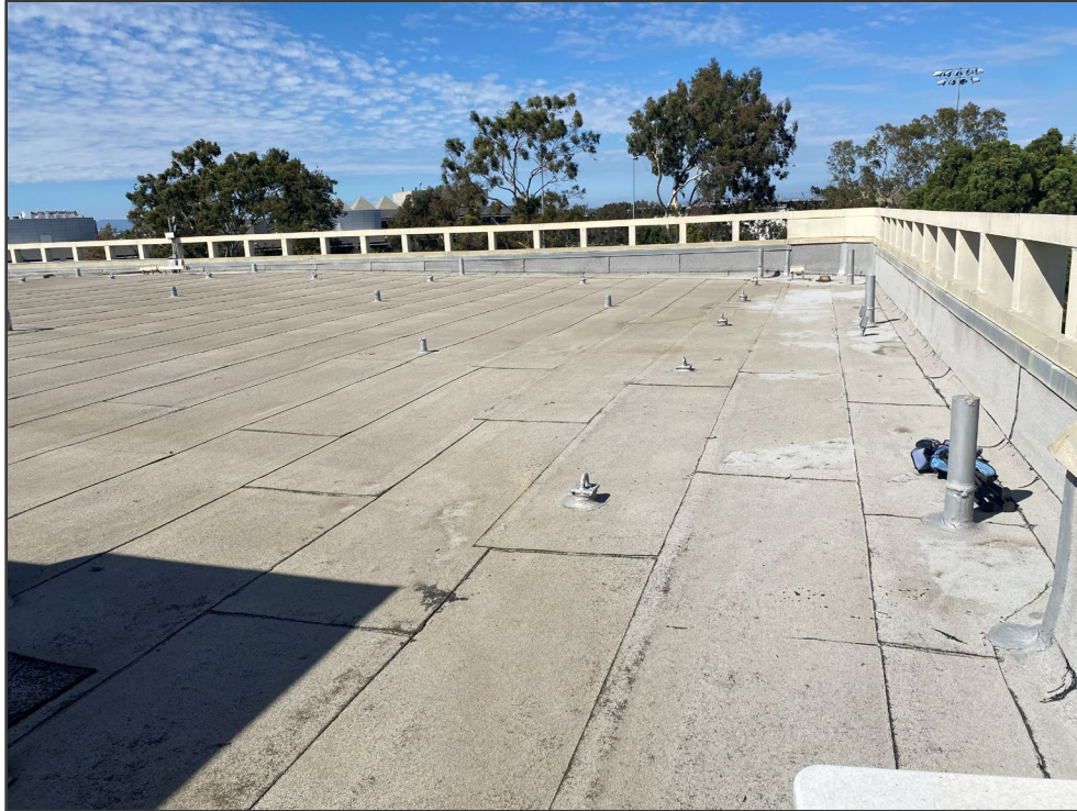
Figure 41 Existing Asphalt Membrane Roof
