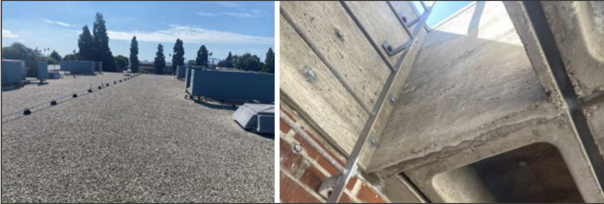
Figure 7 Existing Concrete Roof with Gravel Coating
