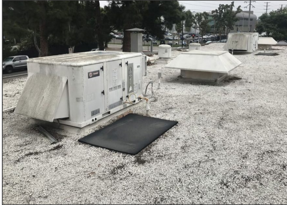
Figure 16 Existing Built up Roof with Gravel Coating on Top
