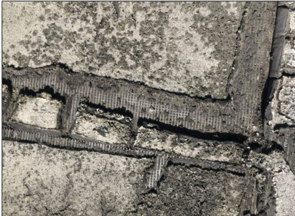
Figure 26 Existing Roof Condition
