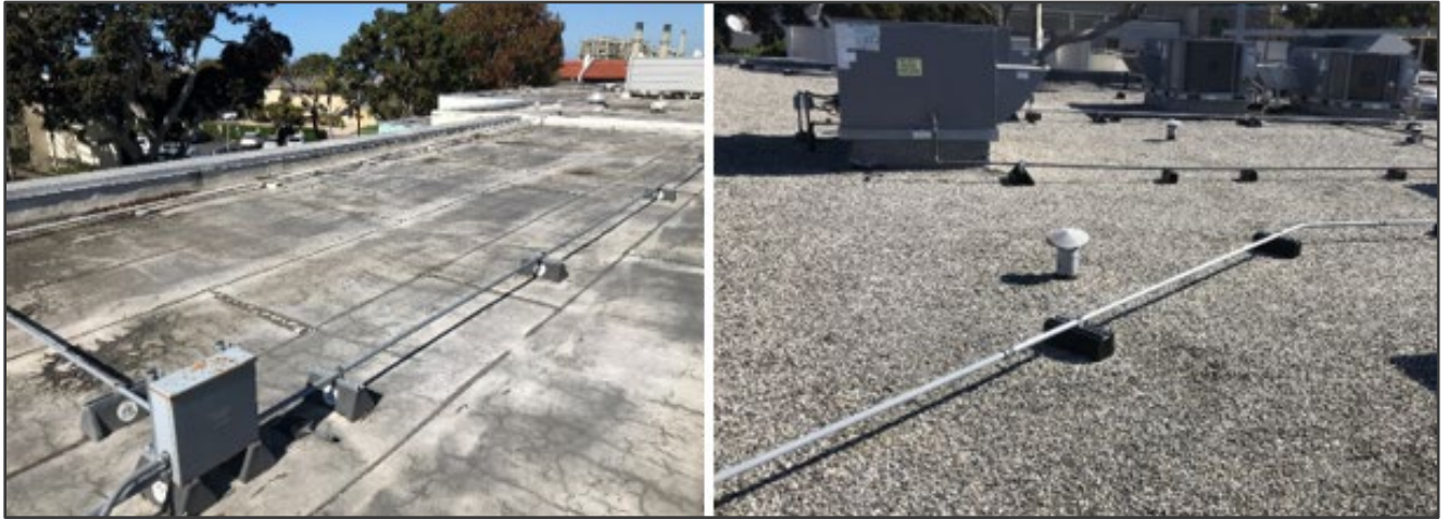
Figure 25 Existing Asphalt (left) and Built-Up Roof with Gravel (Right)
