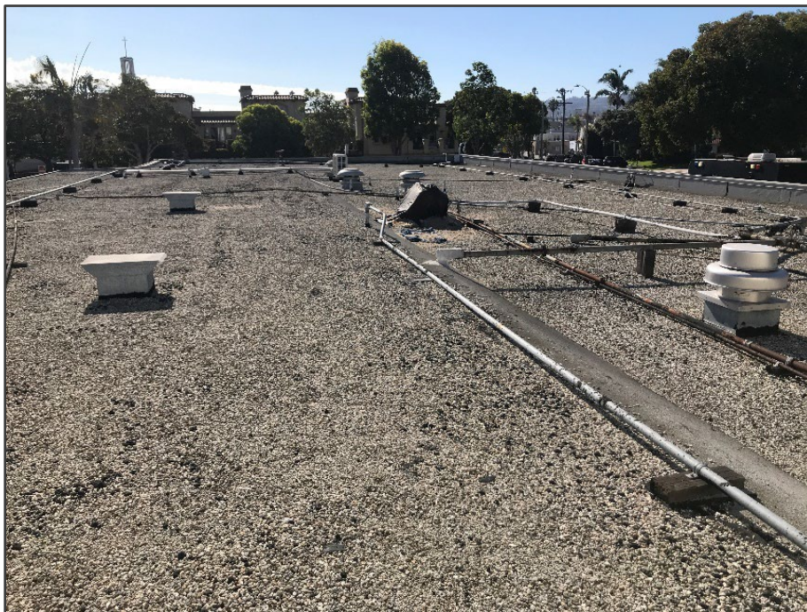
Figure 32 Existing Built-Up Roof with Gravel
