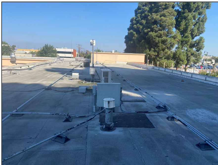
Figure 5 Existing Modified Bitumen Roof
