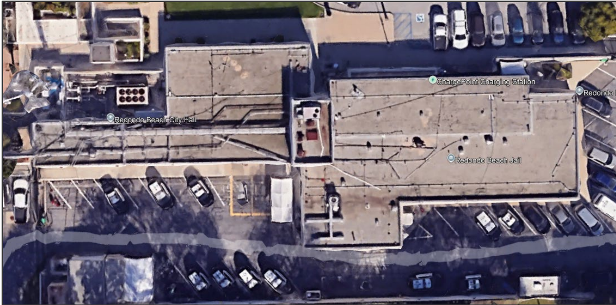
Figure 31 Aerial View of Redondo Beach Civic Center Police Department
