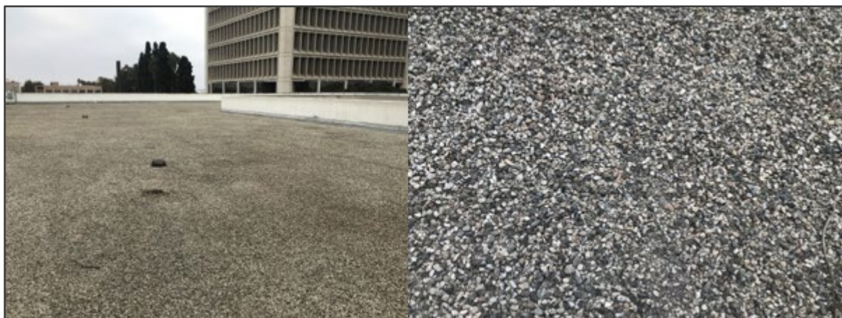
Figure 19 Existing Built up Roof with Gravel Coating on Top
