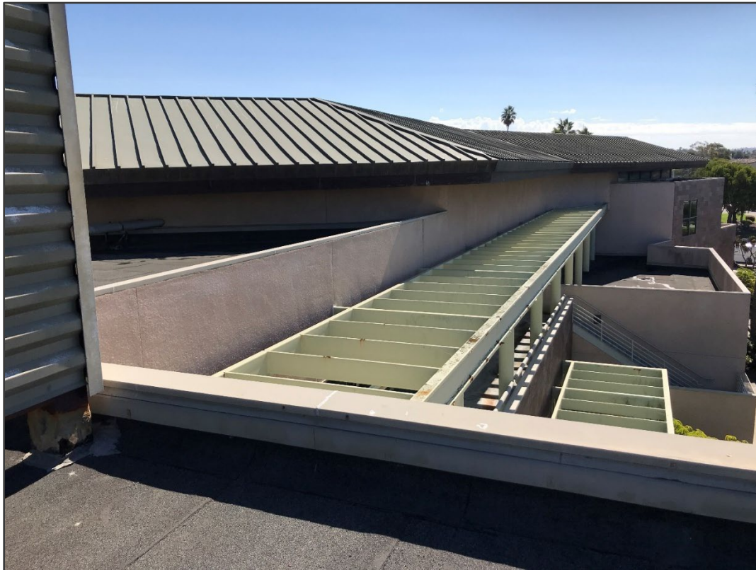
Figure 29 Existing Asphalt and Metal Roof
