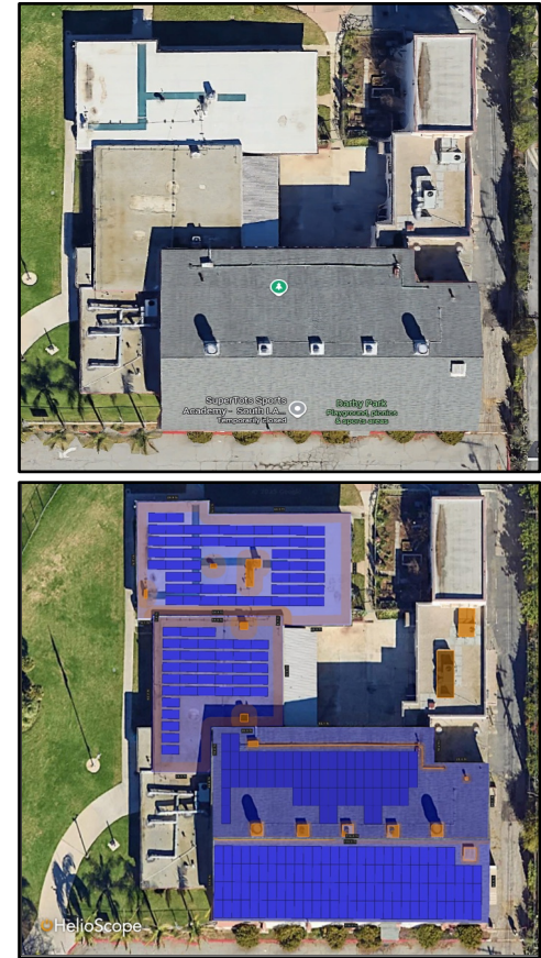
Aerial View (Top Picture) and Rooftop Solar PV (Bottom Picture)
